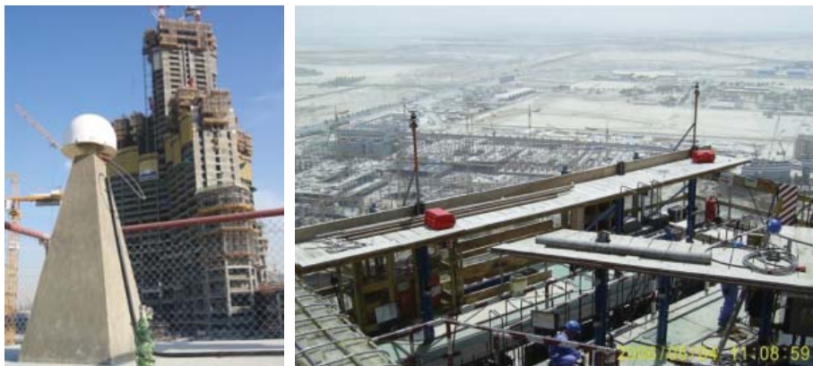
Figure 6. The measurement system, consisting of a reference base station (left) and total station (right), used to triangulate current positions © Samsung C&T
